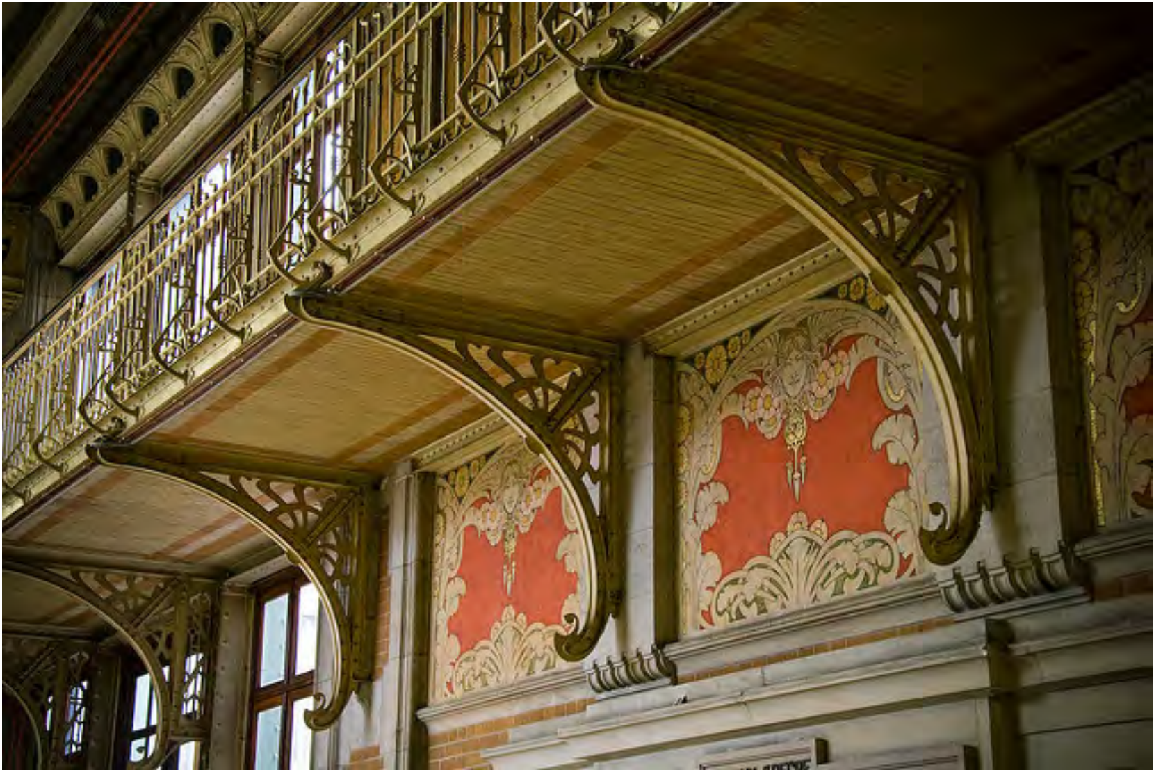
sgraffiti panels by Privat Livemont in indoor playground at Schaerbeek School No 1
