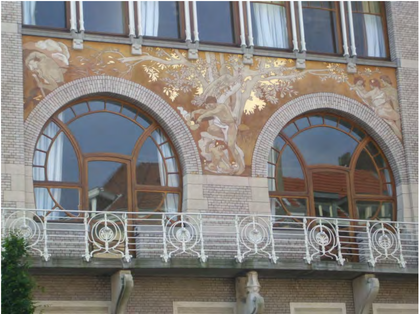
Sgraffiti on facade of Ciamberlani house executed by Adolphe Crespin
