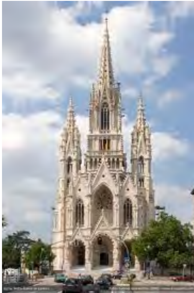
Notre-Dame de Laeken Church, Brussels completed 1872
